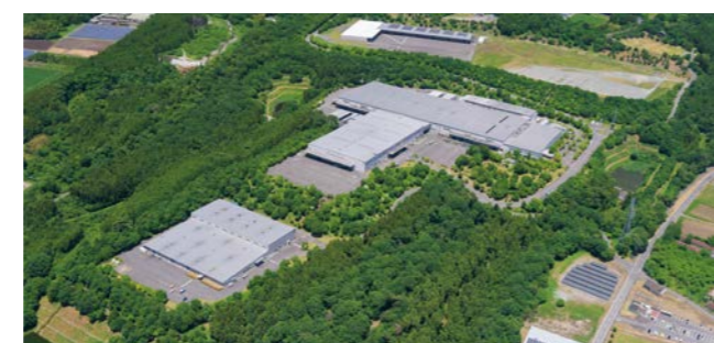
The Sanden Forest/Akagi Plant created using close-to-nature construction methods
